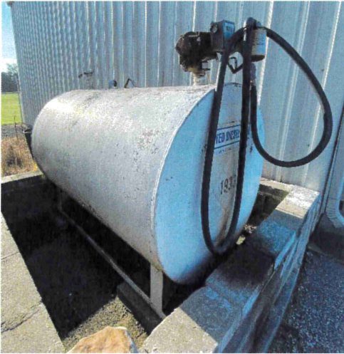
Figure 10: 500-gallon diesel AST
